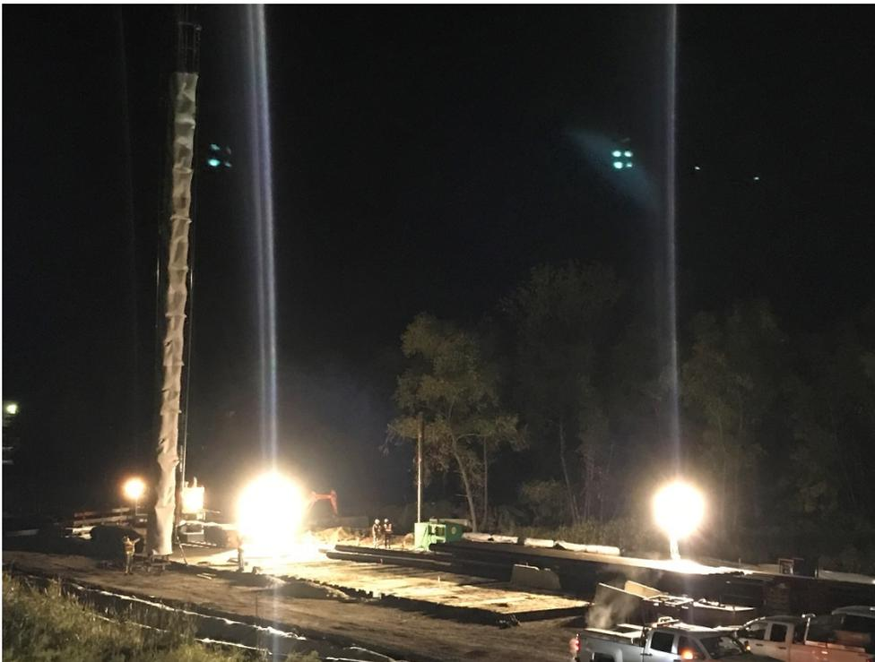
Lights illuminate the job site for safety as crews begin night piling work in Eden Prairie. Crews constructed a sound dampening shroud for the pile driver, as seen towards the left of the image.
