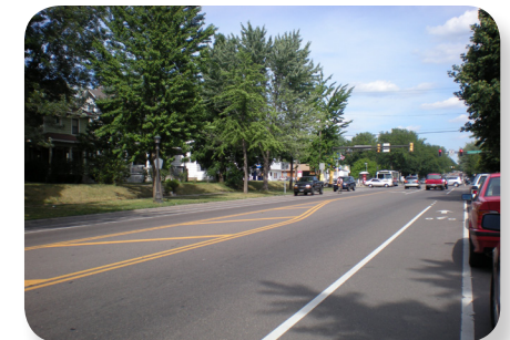
Figure 9-14: Marshall Avenue in St. Paul is a “complete street” with bike lanes, sidewalks, multi-use lanes and bus shelters.
