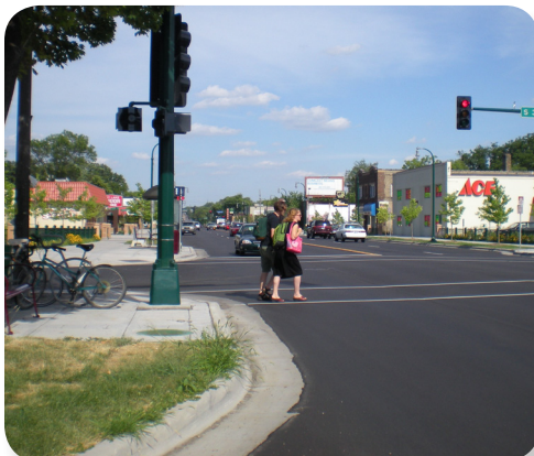
Figure 9-15: Lake Street in Minneapolis includes “bump outs” at crosswalks that shorten the distance pedestrians must be in the crosswalk.
