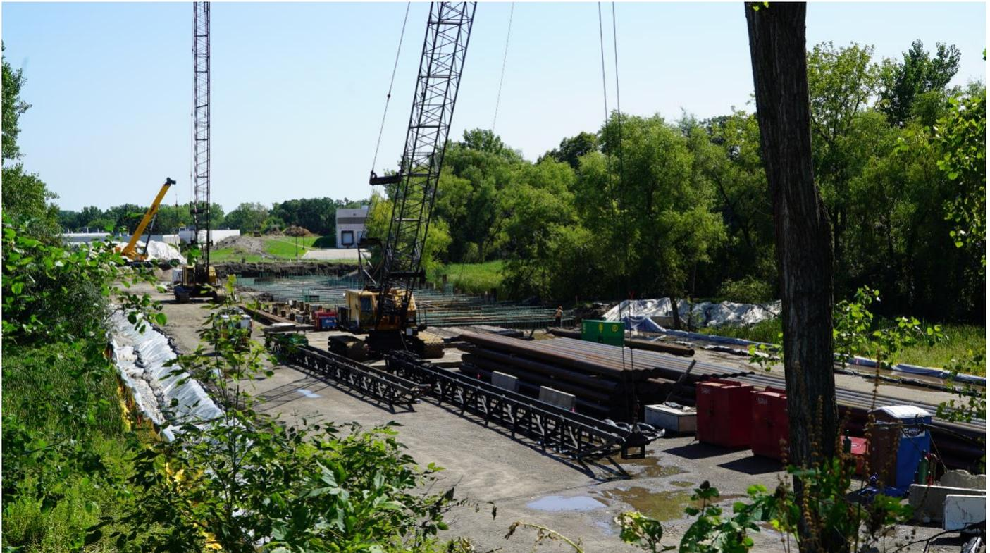
Crews working at the Golden Triangle Station in Eden Prairie to install piles and have started concrete work. Due to vibration sensitive businesses in the area with daytime operations, night piling will begin in early September and will last several months as crews complete work.
