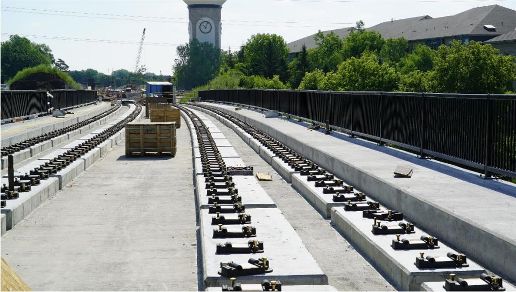
This photo shows what the plinths look like after they are set. The rail for LRT is then pulled across and fixed to the plinths.
