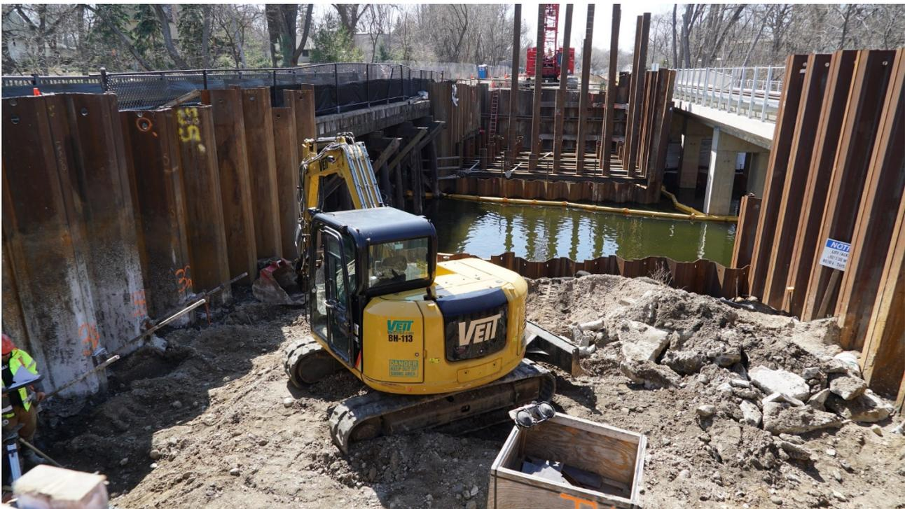
Crews have been working to excavate the abutment for the north end of the Cedar Lake Channel LRT bridge. Piling for this abutment has begun. Piles can be seen in the photo for the south abutment. The new freight bridge is also pictured on the right.
