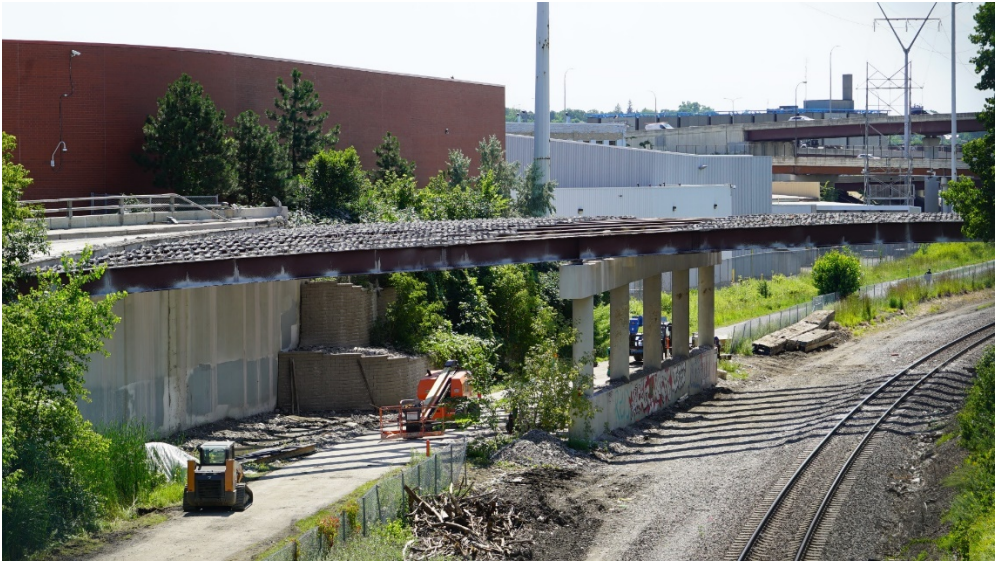
July 2019 A summer photo of Glenwood Bridge demolition.
