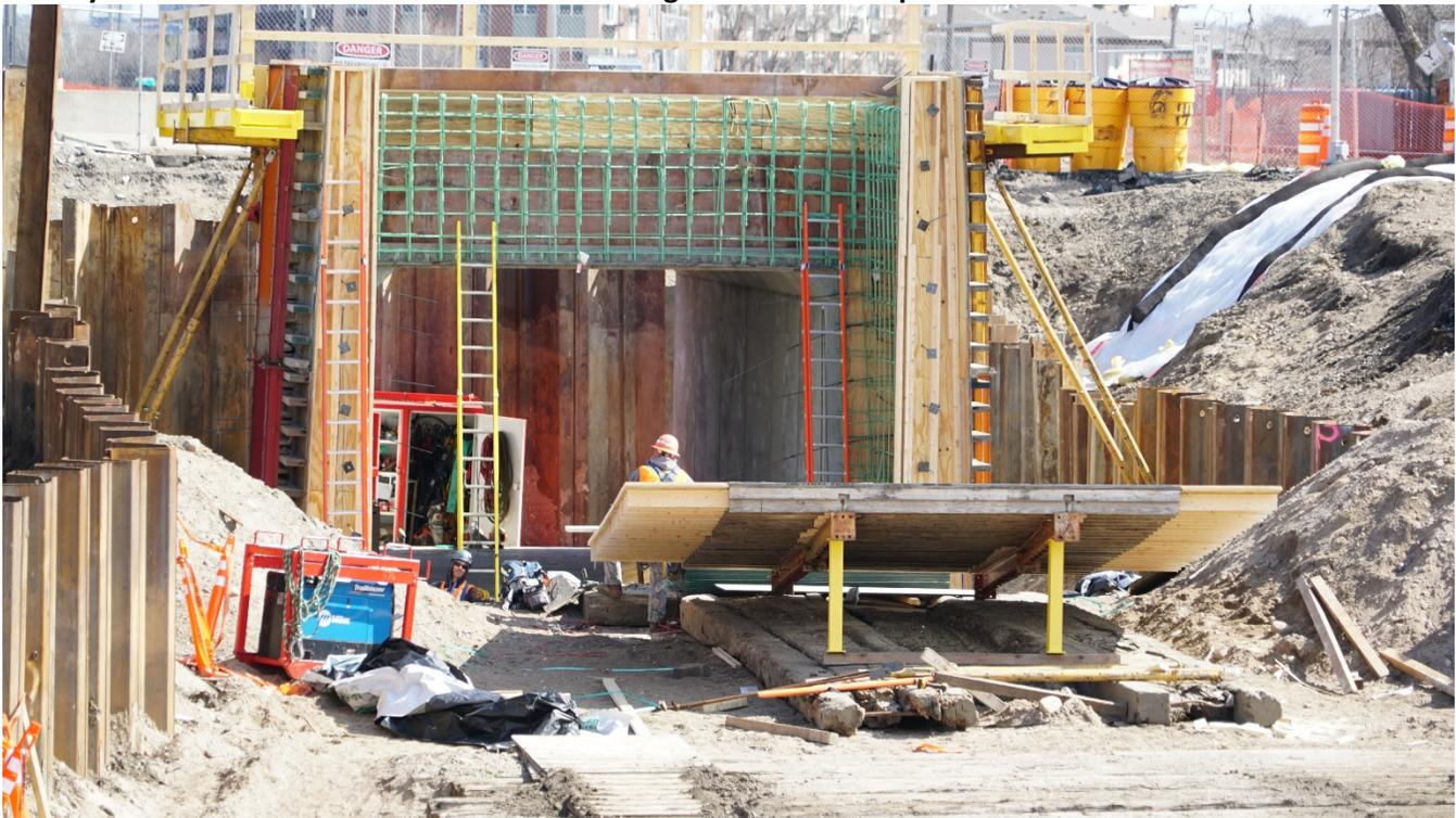
Workers construct the box structure on the approach to what will become the Wooddale underpass. Crews have been conducting piling and excavation work. The work has progressed to a point where we are ready to begin the full closure of Wooddale Avenue on Thursday, April 23 and continue with these activities into the roadway.
