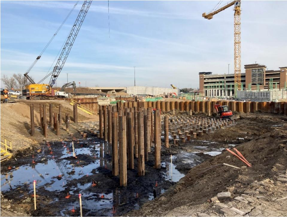
Looking east towards SouthWest Station construction crews install piles that will support the bus loop/roadway. Due to poor soils conditions, project elements including track, stations, roadway and utilities are supported by piles.
