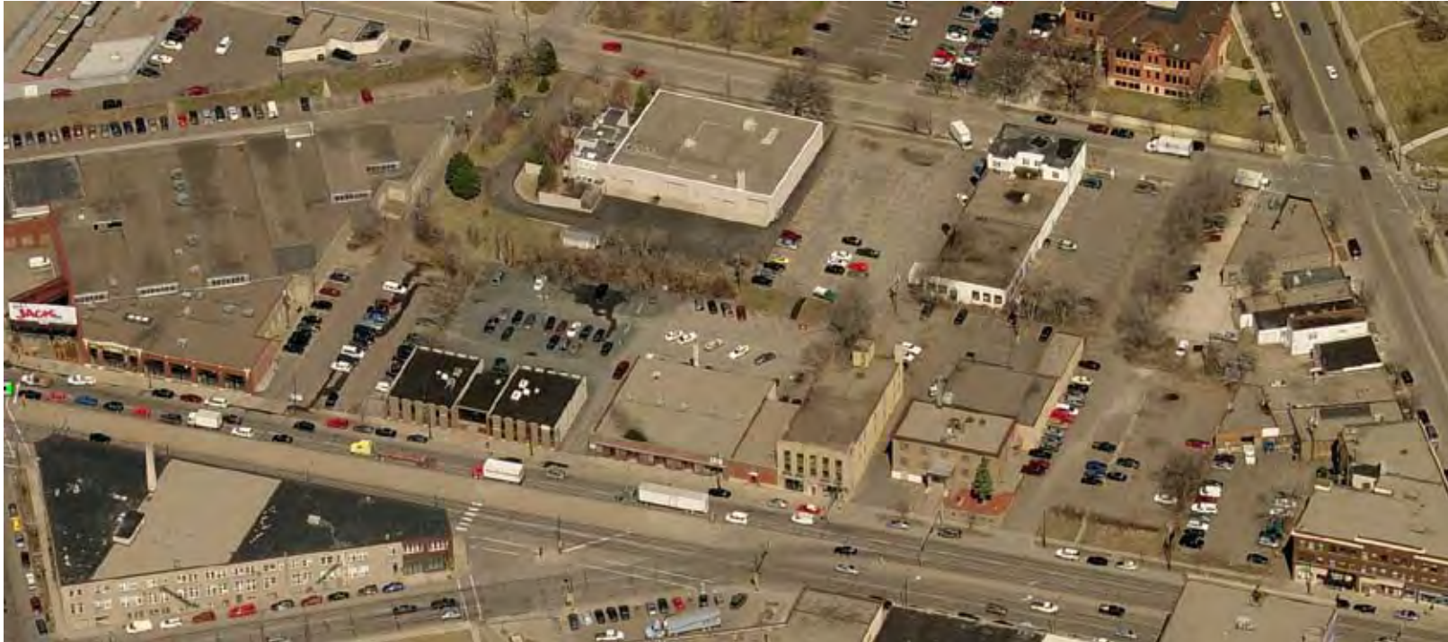
Highway 280 to Raymond Looking North
