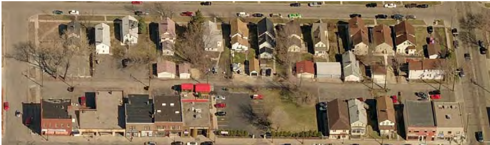
Arundel to Western Looking North
