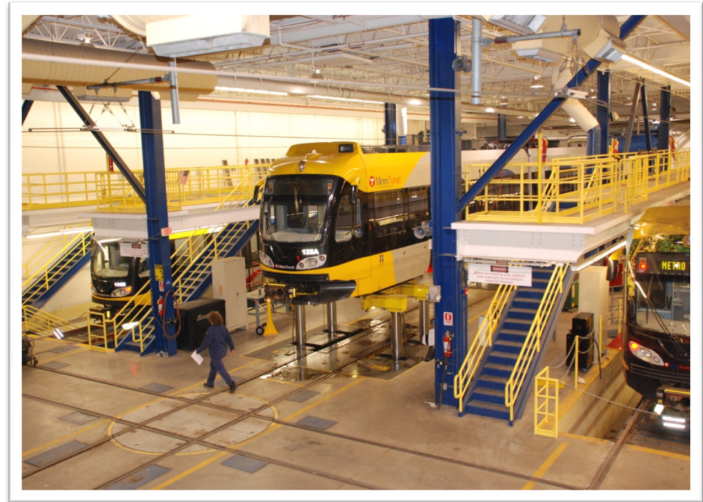
Interior of Blue Line's (Hiawatha) Franklin OMF
