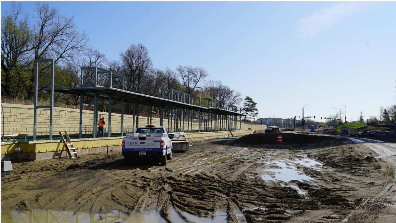
The Eden Prairie Town Center Station is taking shape. Last construction season crews built the retaining walls seen behind the station, allowing station construction to begin.
