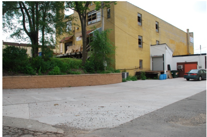
City of St. Paul Neighborhood Commercial Parking Program funds used to build a retaining wall and parking lot for Design Press at 2447 University Avenue
