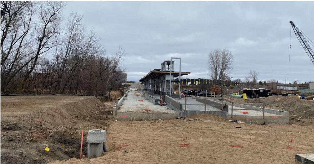
LRT bridge at 212 and Shady Oak: pier work is ongoing, followed by span placement and deck work.
