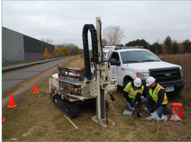
Above left: Crews conducted soil borings and took water samples in late October along the LRT alignment east of Highway 100 in St. Louis Park. Above right: In November, crews excavated test trenches.
