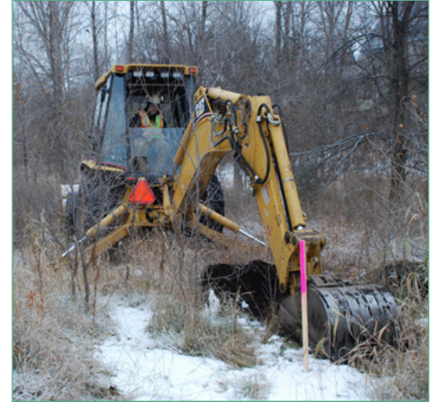
Above left: Crews conducted soil borings and took water samples in late October along the LRT alignment east of Highway 100 in St. Louis Park. Above right: In November, crews excavated test trenches.
