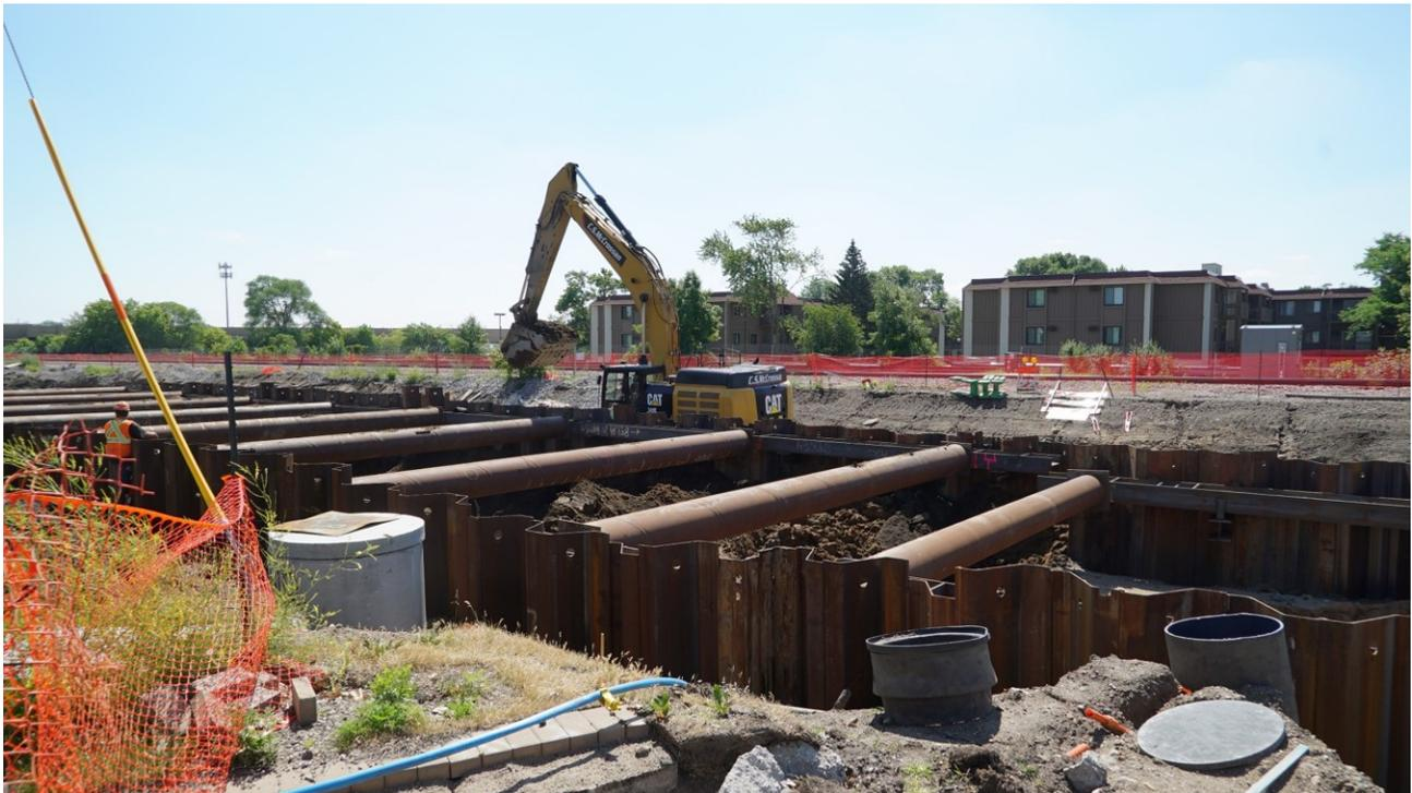
With one half of the Blake Regional Trail underpass constructed on the west, crews are working to build the eastern half. Sheeting has been installed to support the excavation activities. Once excavation activities are complete, crews will advance tunnel construction.
