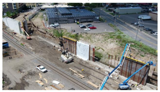
When the project is complete, Southwest LRT trains will cross Glenwood Avenue on a bridge at grade with cars and pedestrians. In order to make that happen, three bridges need to be constructed over the freight rail
