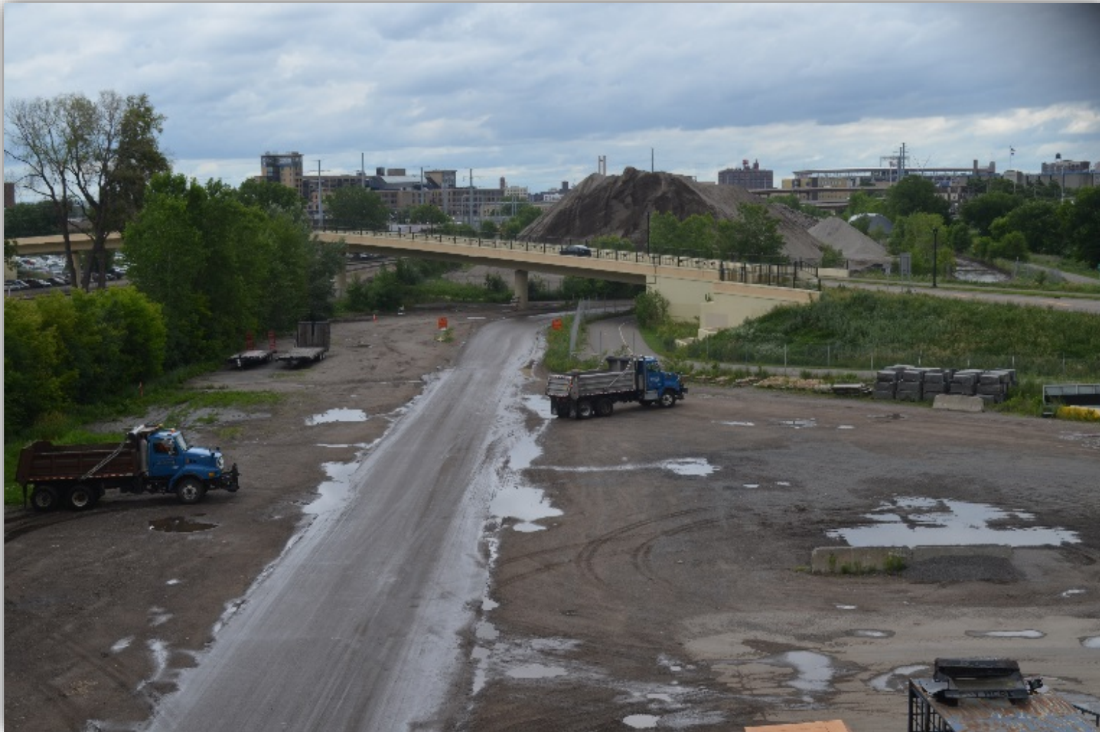
Linden Yards – looking northwest toward the Van White Memorial Blvd bridge
