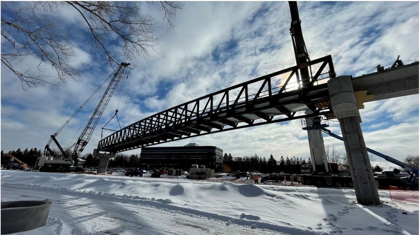
Crews placed the bridge span for the Beltline Boulevard regional trail bridge over the freight rail tracks this past week. [Watch](#) a time-lapse video of crews setting the span.
