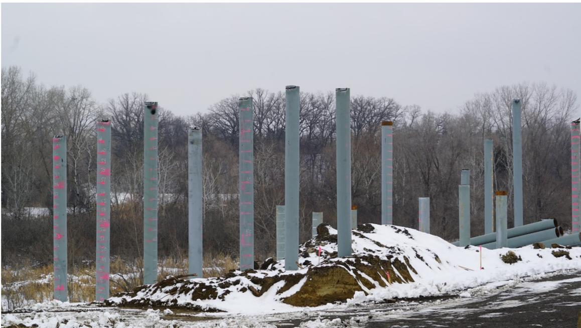
Work to install piles to support LRT infrastructure is ongoing in the area. Piles are driven into the ground until they reach the proper depth and then are cut-off to the appropriate height.
