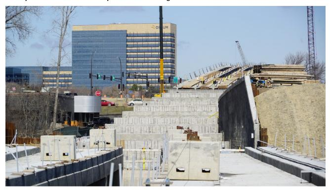
With bridge beams recently placed, crews work to advance the deck of the Shady Oak LRT bridge in Eden Prairie. Looking north from the Golden Triangle Station.
