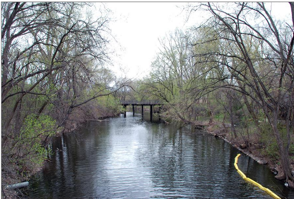
Figure 43. Between the bridges, facing southeast from Bridge No. 6
