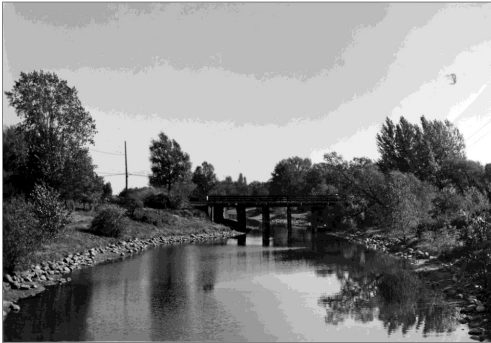
Figure 19. Kenilworth Lagoon and Bridge No. 5, 1936 (Minnesota Historical Society Collection)
