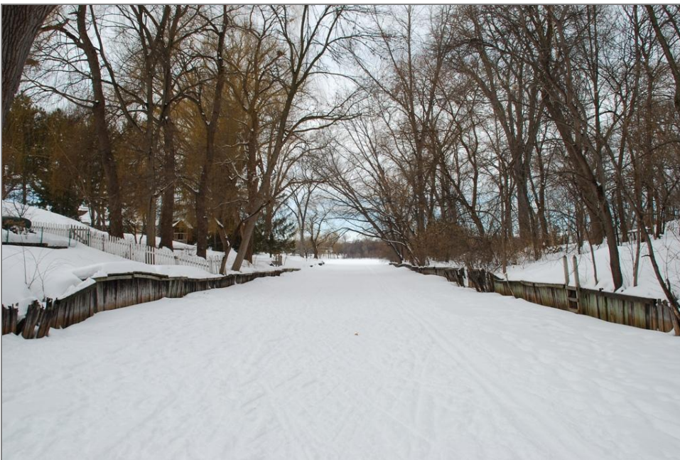
Figure 71. WPA Wood Pile Channel Walls/Breakwaters, facing northwest
