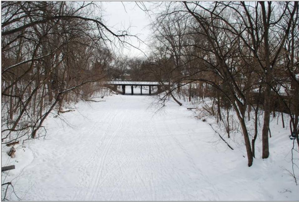
Figure 42. Between the bridges, facing southeast from Bridge No. 6
