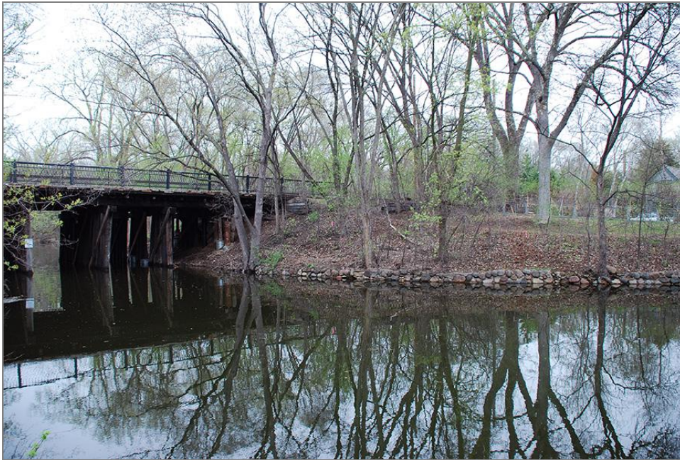
Figure 68. WPA Rustic Style Retaining Wall, north shore of lagoon, facing north
