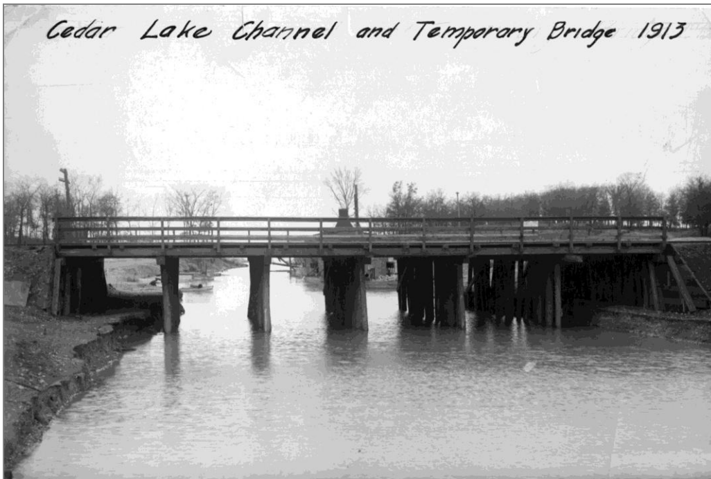
Figure 16. Bridge No. 5, 1913 (MPRB, Minnesota Historical Society Collection)
