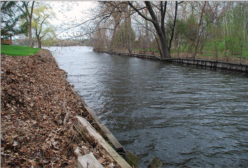
Figure 47. Channel from south shore, facing northeast
