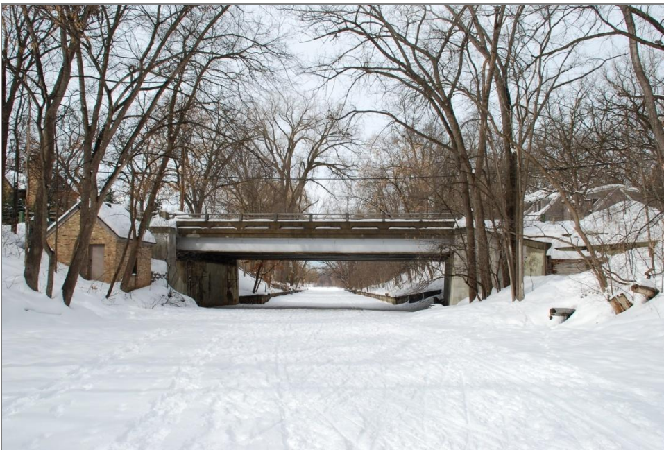
Figure 39. Area between the bridges, with Bridge No. 6 in the distance, facing northwest
