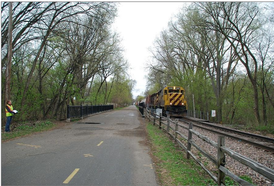
Figure 55. Kenilworth Trail and the M&StL/TC&W railroad line passing over Bridge No. 5, facing southwest
