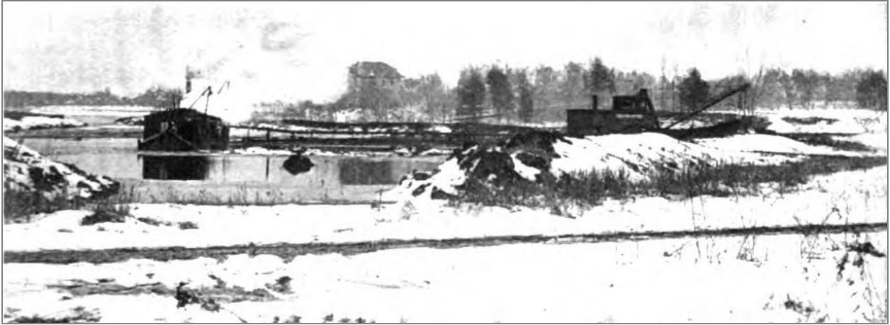
Figure 5. Hydraulic and Orange Peel Dredges at Work in the Lagoon between Lake of the Isles and Cedar Lake (MBPC 1910:35)
