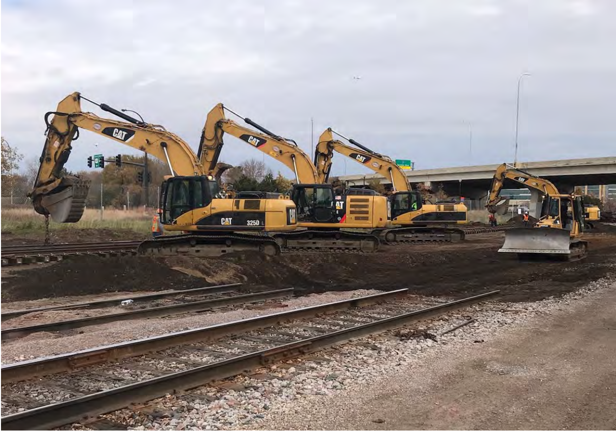
Synchronized excavators shift the freight rail track near Excelsior Boulevard.
