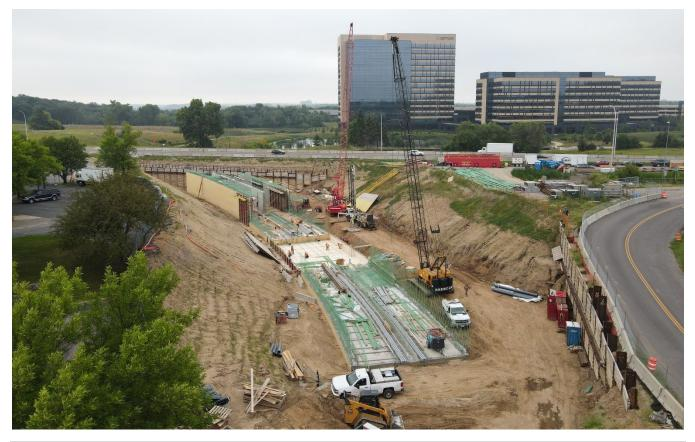
The construction of the LRT tunnel under Highway 62 is a multi-year process. With traffic shifted onto one side of the Highway crews have built the base of the tunnel are are working to progress walls and roofing.
