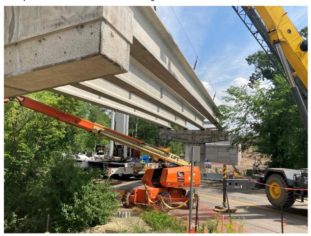
Bridge beams are set into place for the Nine Mile Creek Bridge in Eden Prairie. One of the many bridges currently in construction, the bridge crosses over both Nine Mile Creek and Flying Cloud Drive (pictured) to connect to the Golden Triangle Station. Work will continue through 2021 to construct the bridge deck.
