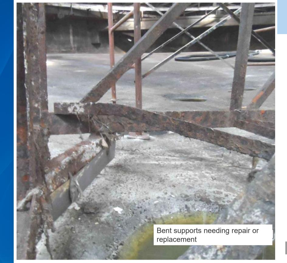
Mounting hardware, steel supports and normal wear parts need to be inspected and replaced, all internal surfaces need sand blasting and protective coatings applied
