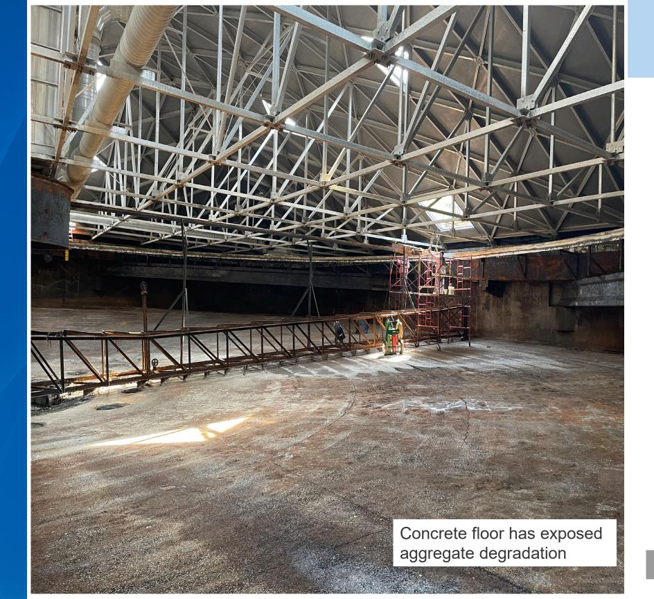
The steel and concrete structures inside a primary tank are immersed and operate in a very harsh environment
