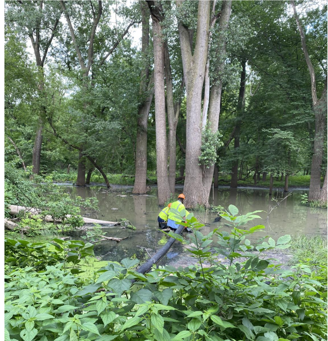
Operations staff setting up pumping
