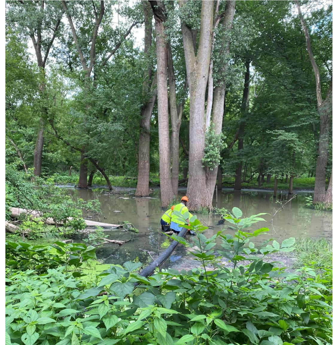
Operations staff setting up pumping
