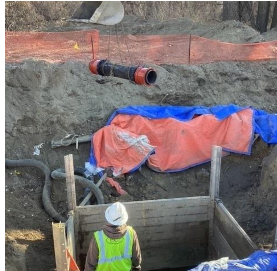
Pipe Segment Replacement
