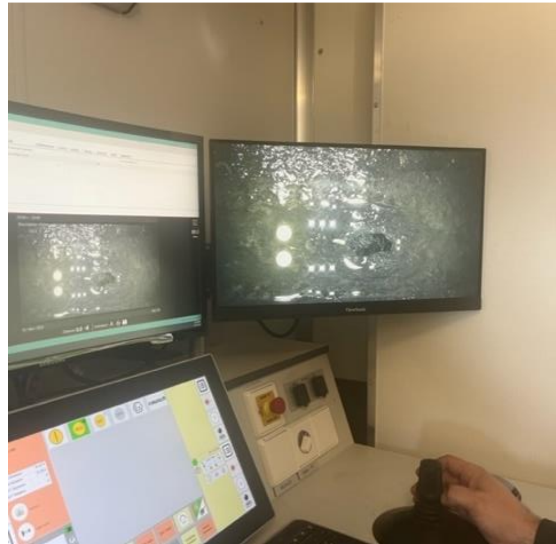
CCTV Inspection – Additional Holes
