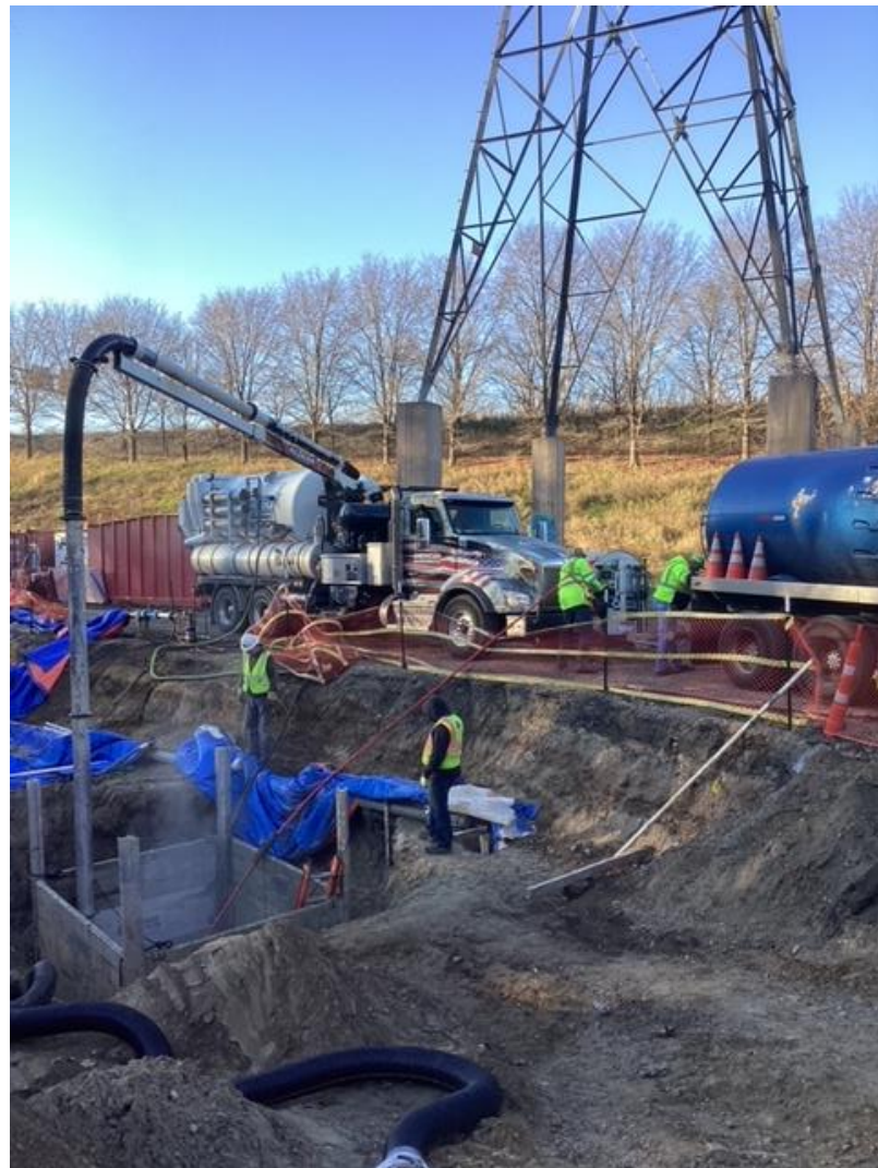
Repair and Cleaning Operation
