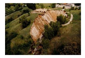
Figure 2: Interceptor failure - Minnesota River
