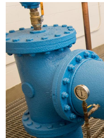
Example of pipe coated with an insulative coating
