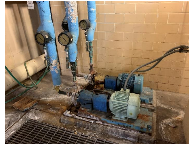
Booster pumps P647 and P648 to be removed.
