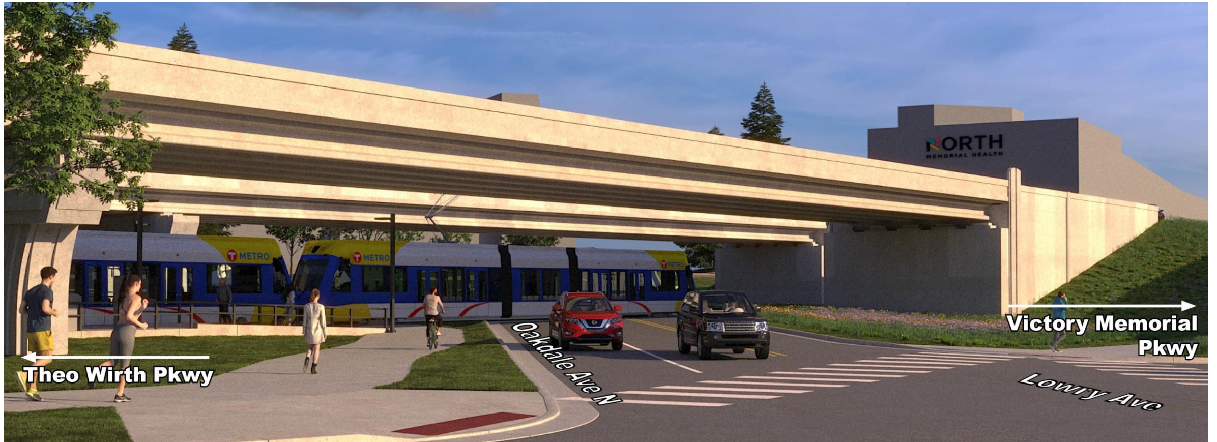
Intersection of Theodore Wirth Pkwy and Lowry Ave Looking West
