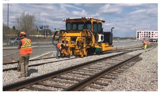
Crews tamp ballast and install ties to shift freight rail to its new alignment during a freight rail outage on April 18.
