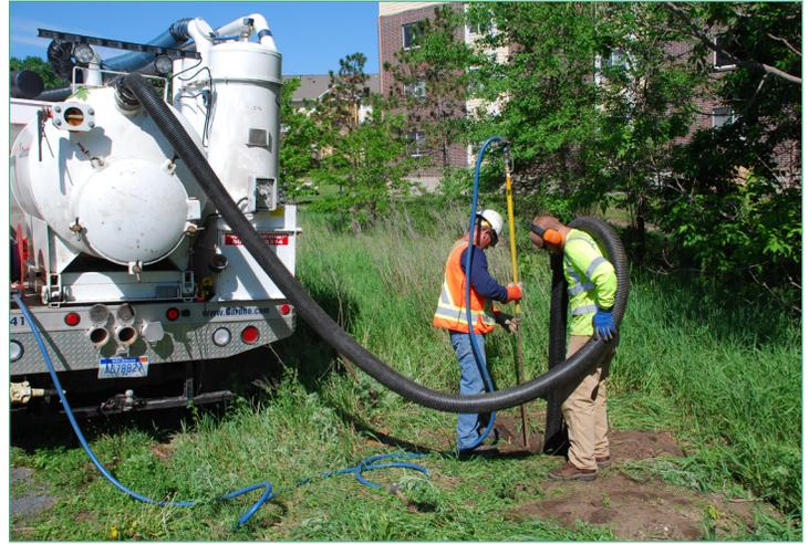
*Above: Crews dig potholes in early June near Highway 100 in St. Louis Park as part of subsurface utility engineering to locate water lines for the Southwest LRT Project.*
