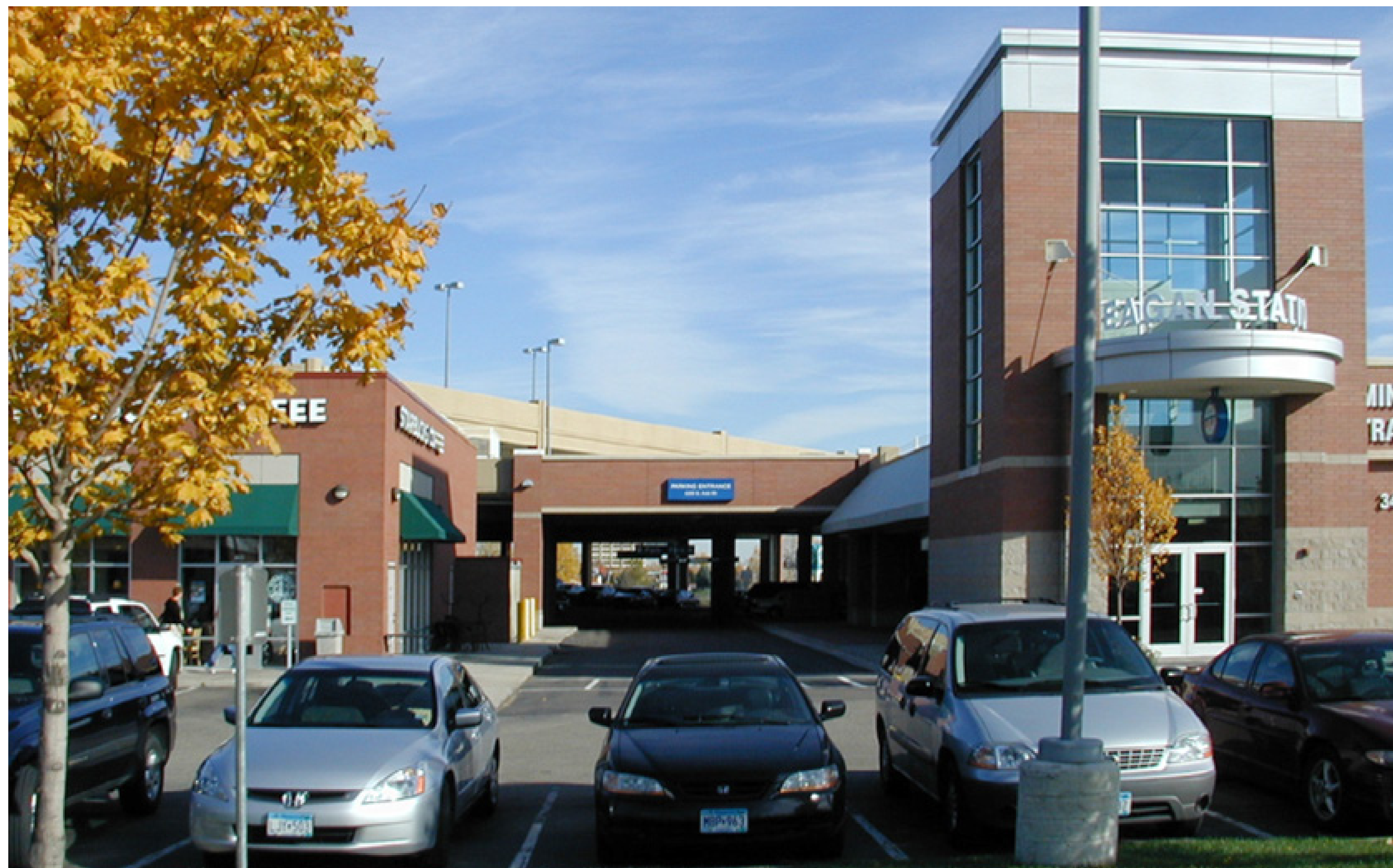
Eagan Transit Center - A 3-level park-and-ride facility and bus passenger terminal co-located with retail uses in Eagan, MN
