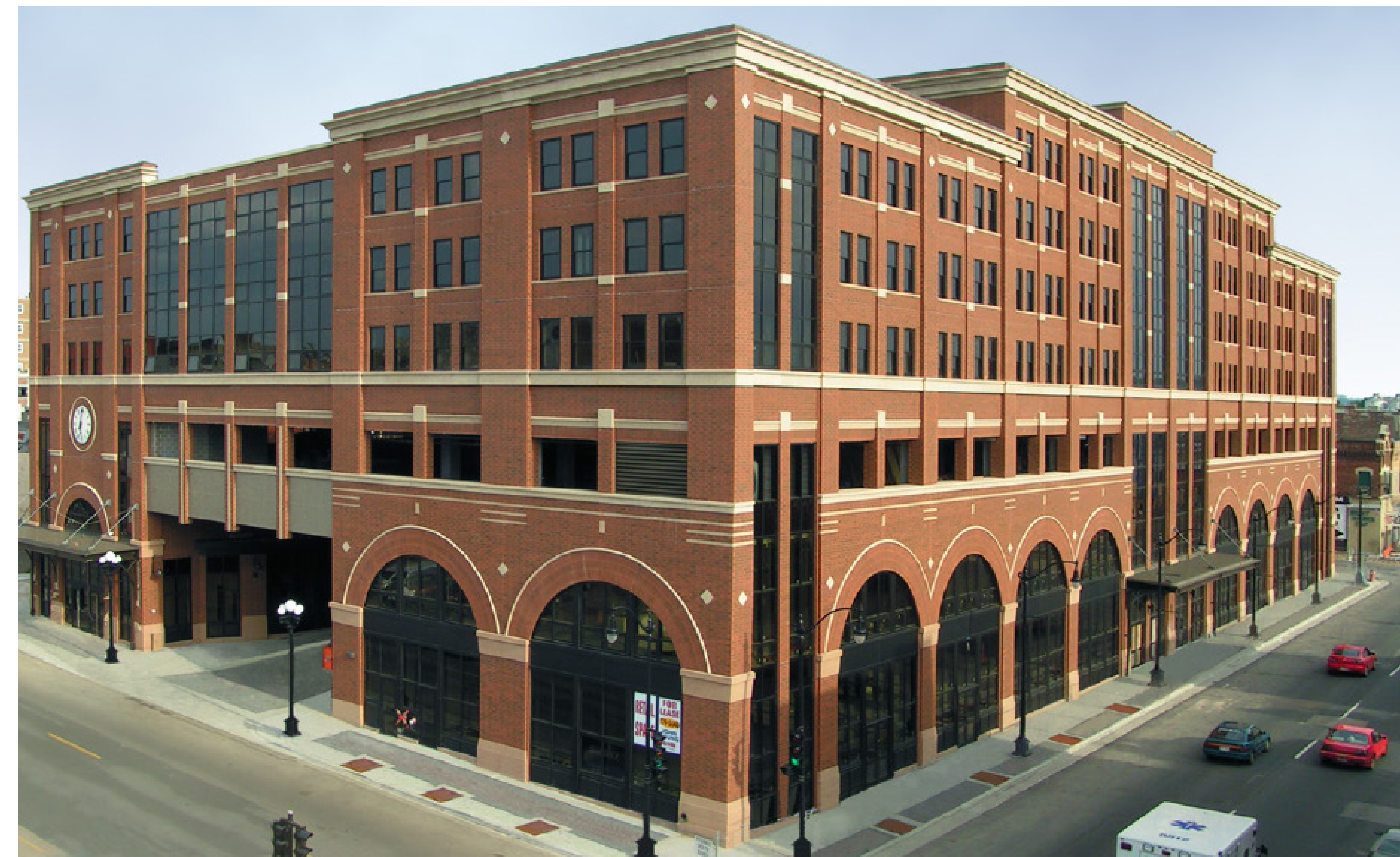
Grand River Station - Bus facility, parking, retail, housing, and office in La Crosse, WI
