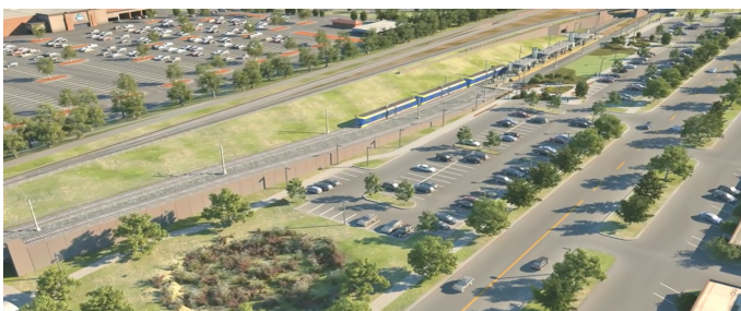
Louisiana Avenue Station
