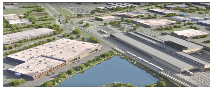
Operations and maintenance facility at Shady Oak Station
