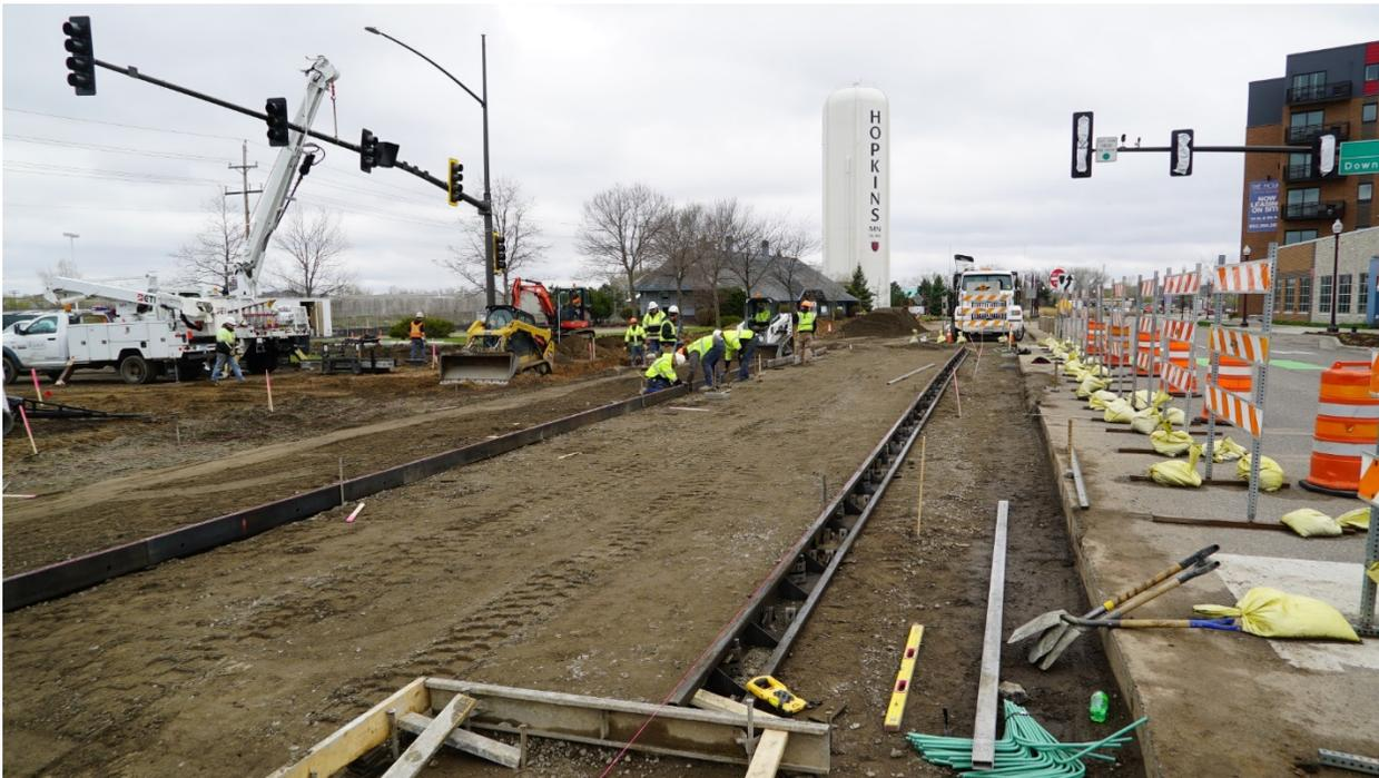
Crews reconstruct 8<sup>th</sup> Avenue in Hopkins to accommodate an LRT crossing. Crews are working to set forms for concrete panels.
