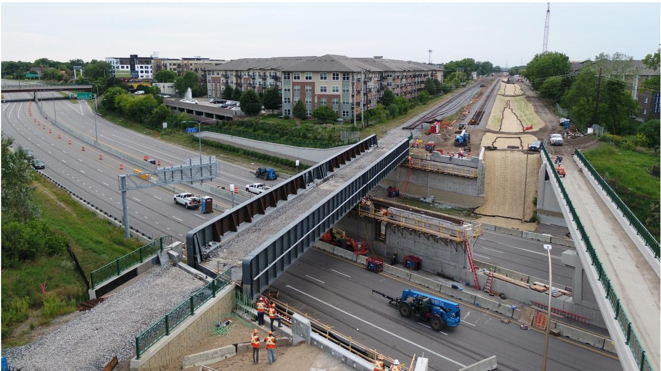
The freight railroad bridge is just starting to be pulled off of its old abutments and shifted to its new permanent location. Moving the bridge took a fraction of the time intended due to its excellent design and advanced construction planning. [Watch the full bridge move here.](#)
