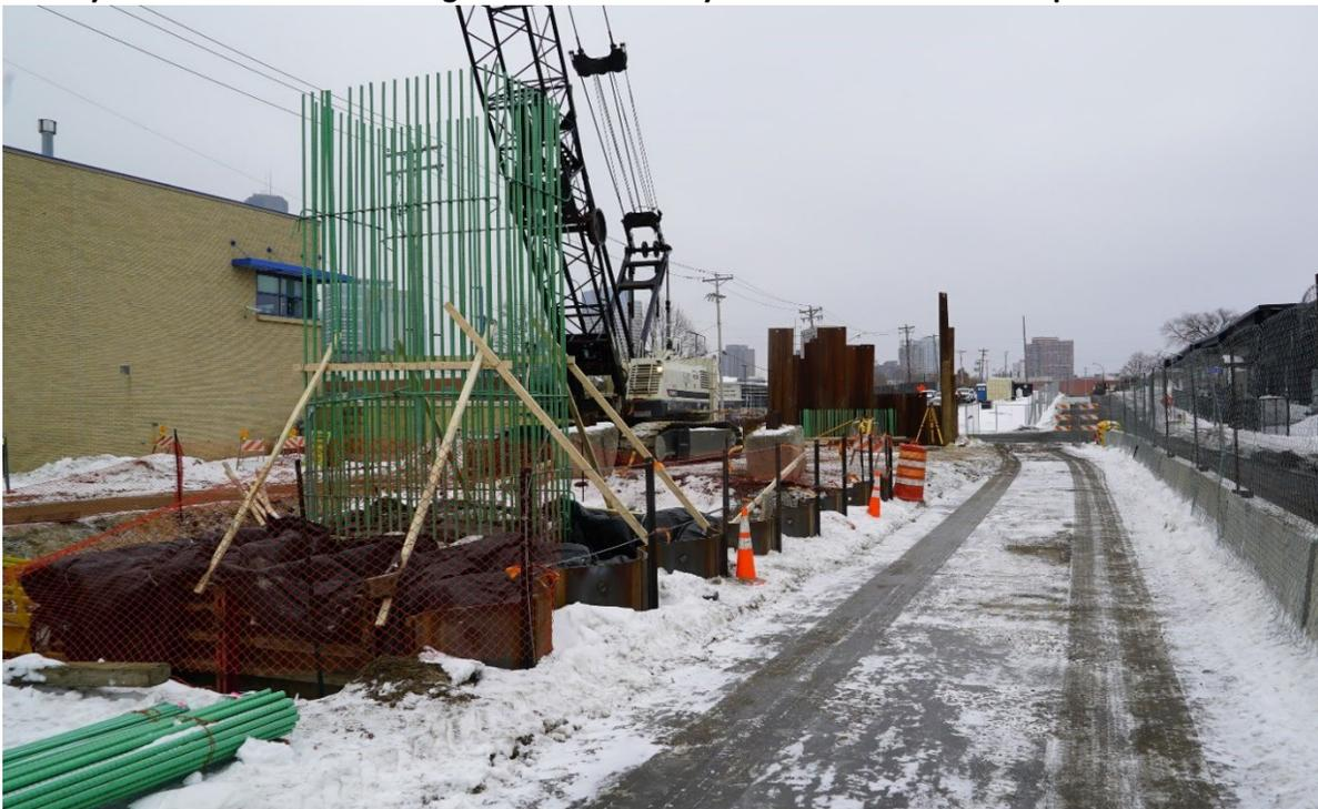
Progress is being made on the LRT bridge spanning from Royalston Avenue over North 5<sup>th</sup> Avenue and North 7<sup>th</sup> Street. Crews are working on the bridge piers and abutments, with intermittent pile driving in the area.
