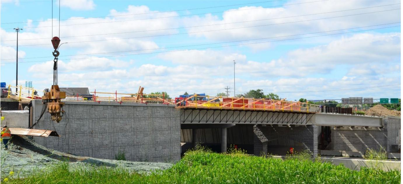
With beams already set-in place crews are advancing bridge deck construction for the I-494 Bridge at Flying Cloud Drive in Eden Prairie. Crews build forms in the daytime while the majority of concrete is poured at night during a road closure.
