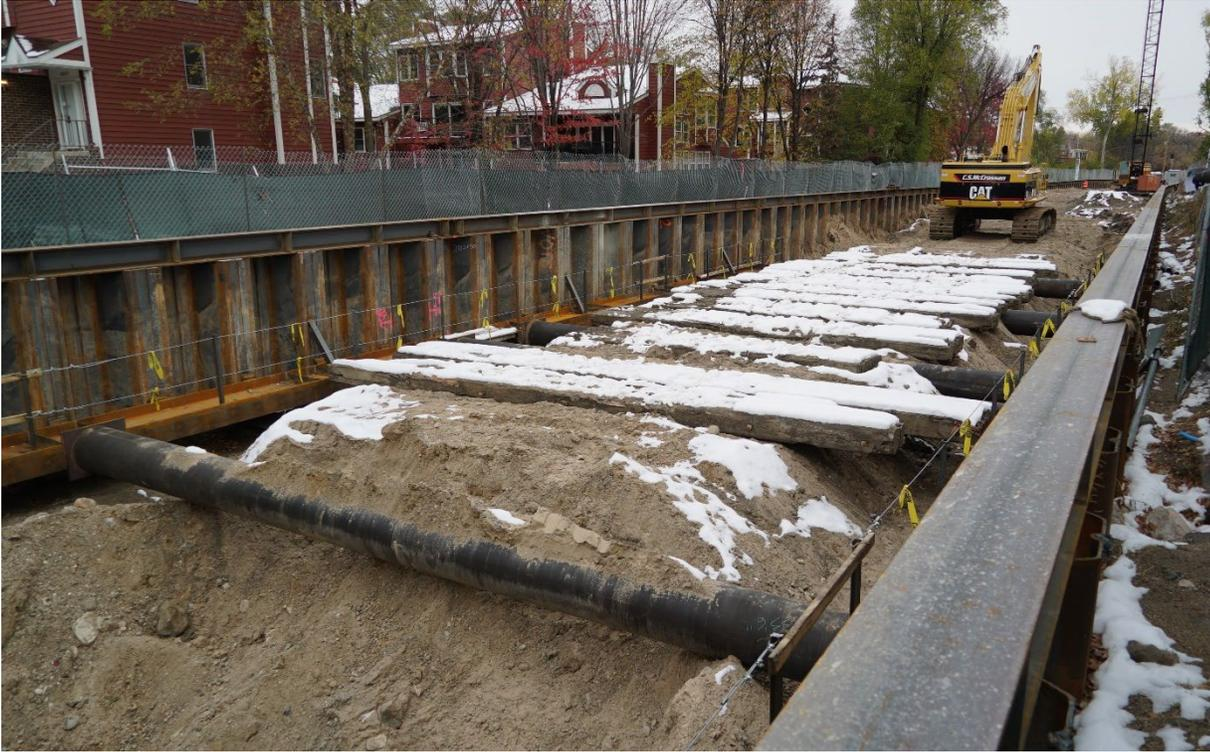
The construction of the Kenilworth tunnel is progressing with a cell-by-cell excavation approach, where 100 feet are excavated at a time. Once sufficient depth is reached, concrete work begins. Specialized equipment is being brought into the corridor to help with excavation.
