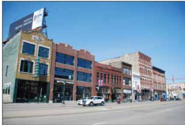
Minneapolis Warehouse Historic District
