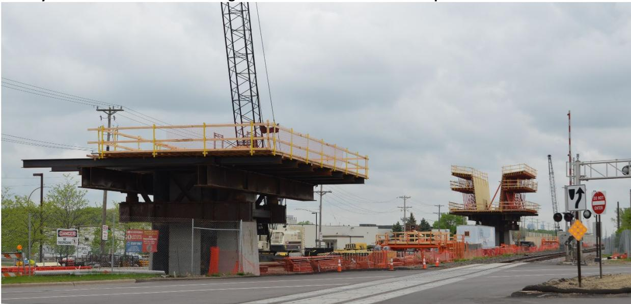
With the LRT bridge piers nearing completion, the structural forms to take the bridge over the roadway and freight rail are starting to take shape. The form work in the front image is called a pier table, which taken quite literally means the base or “table” for the bridge to be placed on the piers. The bridge structure is a post-tensioning box girder. This type of bridge can efficiently span long distances. The initial shape of the box girder is visible on the second pier in the background.
