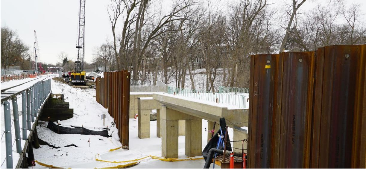
Crews are working on the final pier and completing abutment work for the Cedar Lake Channel freight bridge, with final span work to follow. Once the new freight rail bridge is completed in the spring, the old freight rail bridge will be removed, and a new LRT bridge will be built.
