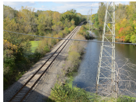
Wetlands adjacent to BNSF Line
