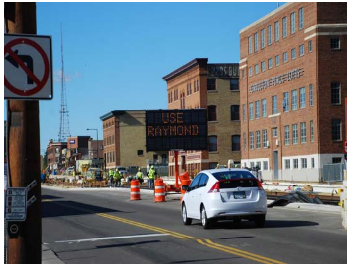
VMS used to alert drivers to closures of University Avenue intersections during the fall of 2011
