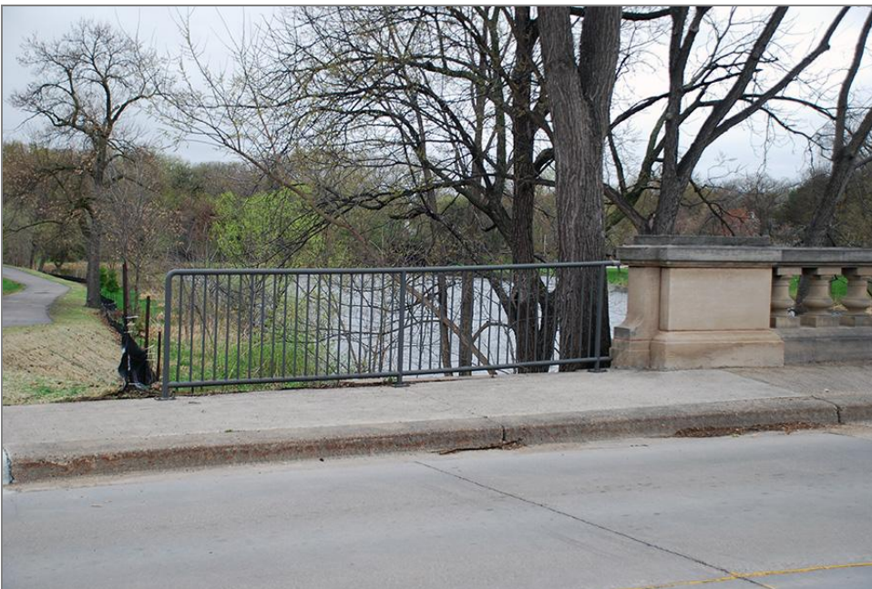
Figure 81. Tube Steel Railing located at the west side of the south end of Bridge No. 4, facing northwest
