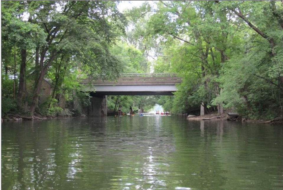
Figure 38. Area between the bridges, with Bridge No. 6 in the distance, facing northwest
