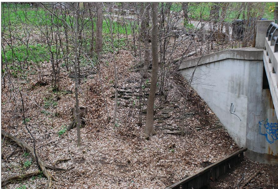
Figure 76. Stone retaining wall located on the northwest corner of Bridge No. 6, facing northeast
