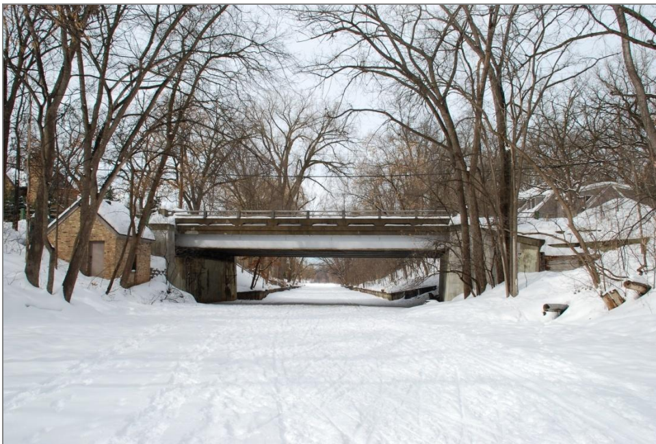
Figure 39. Area between the bridges, with Bridge No. 6 in the distance, facing northwest
