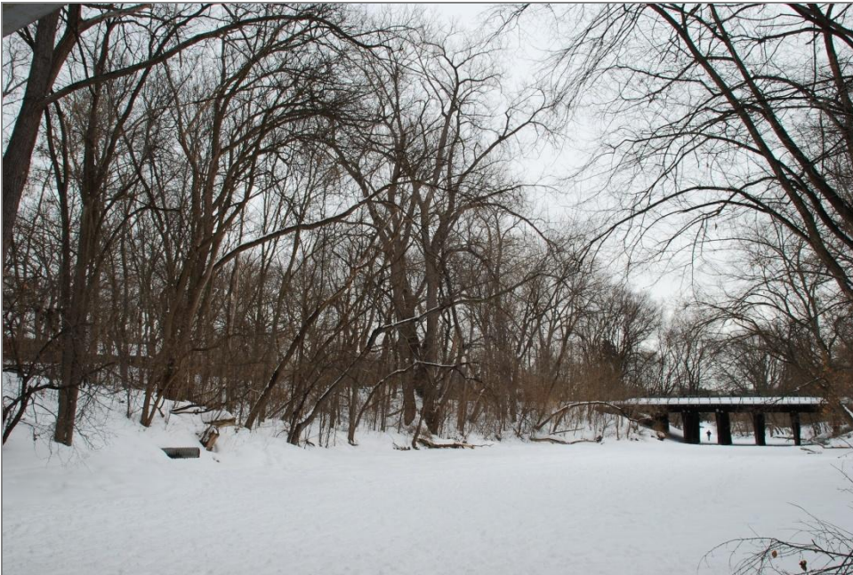
Figure 40. Area between the bridges, with Bridge No. 5 in the distance, facing east
