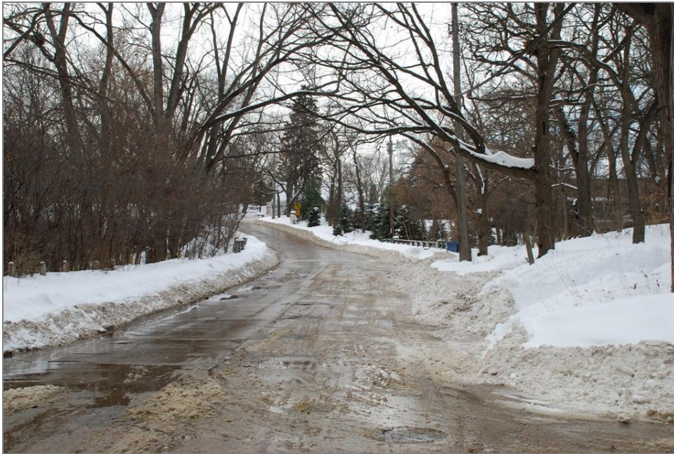
Figure 54. Burnham Road as it passed over the Kenilworth Lagoon/Channel, facing southwest
