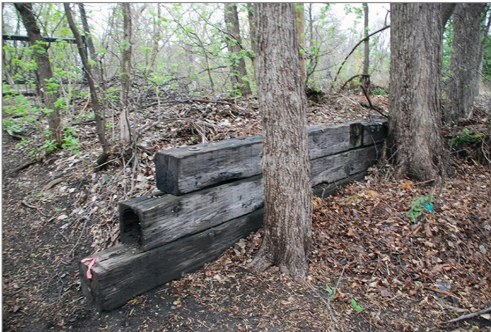
Figure 75. Railroad tie retaining wall, facing northwest
