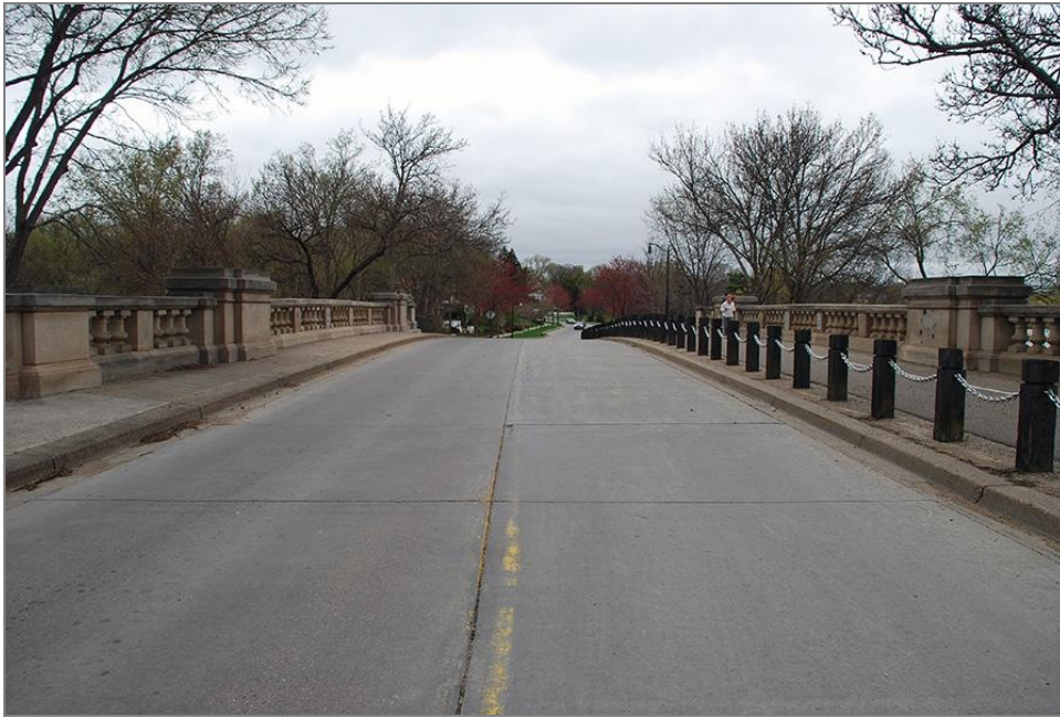
Figure 52. West Lake of the Isles Parkway over Bridge No. 4, facing north
