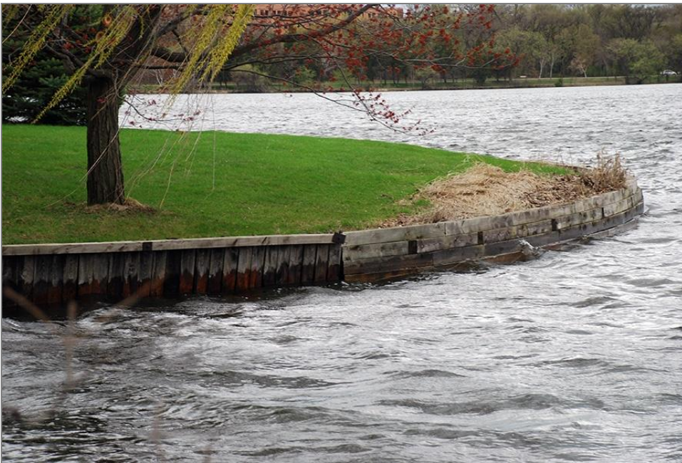
Figure 48. West end of channel at Cedar Lake, facing southwest
