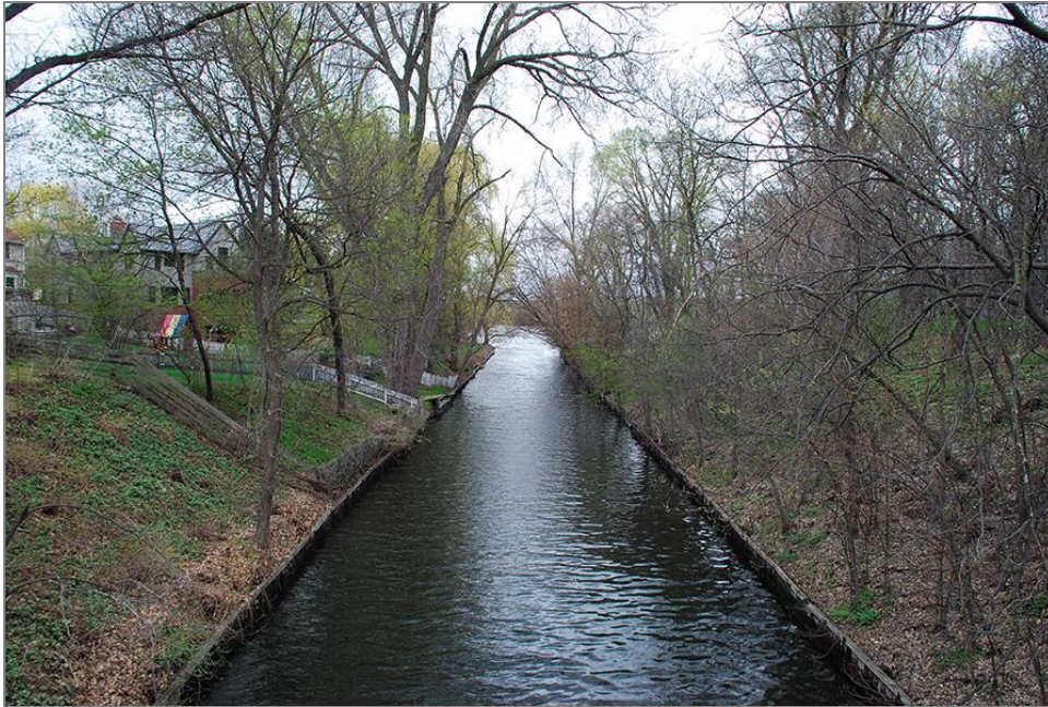
Figure 45. Channel, facing northwest from Bridge No. 6
