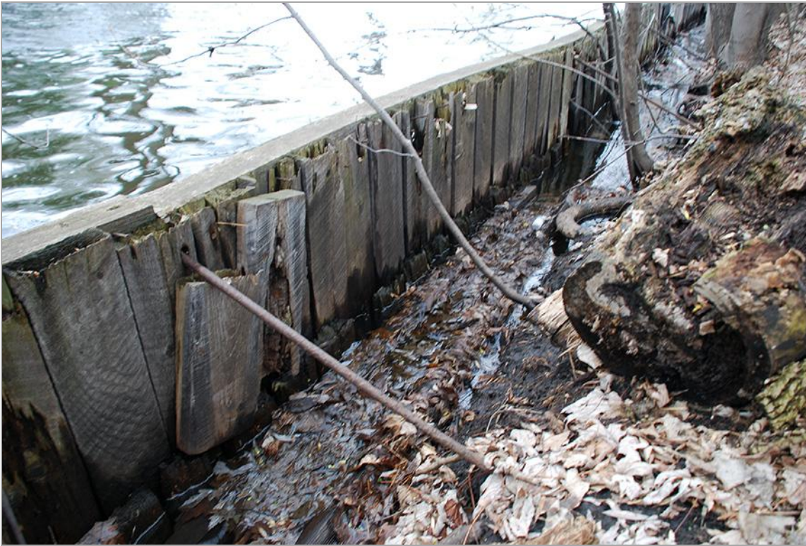
Figure 72. Detail of WPA Wood Pile Channel Wall/Breakwater, showing anchor rod and piles remnants behind current wall, facing southwest
