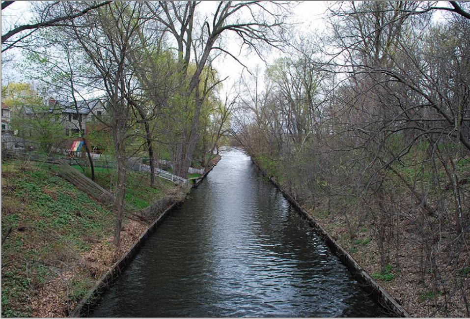
Figure 70. WPA Wood Pile Channel Walls/Breakwaters, from Bridge No. 6, facing northwest
