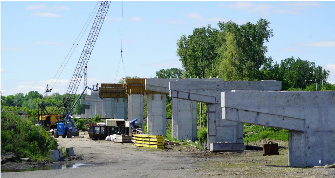
As LRT travels into Hopkins a bridge structure is needed for LRT to cross over freight rail tracks, as seen in the background of this image. The piers for the LRT bridge continue to take shape.
