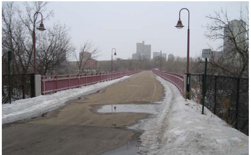
View southwest across Bridge No. 9.
