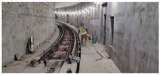
Crews work to install LRT tracks in the Highway 62 tunnel. With the structure complete crews are working to advance the inside of the tunnel. Instead of ballast rock, inside the tunnel the track is directly affixed to the concrete.
