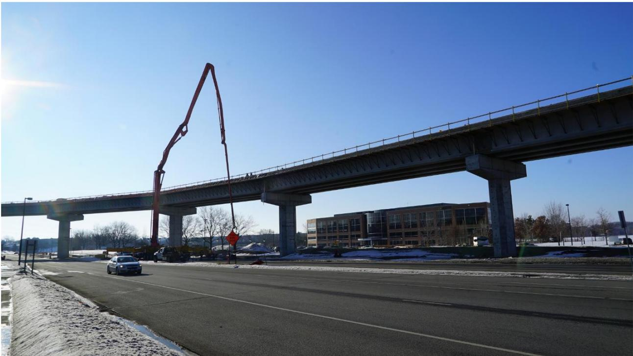
Crews use equipment to place concrete onto the deck of the Prairie Center Drive LRT bridge in Eden Prairie.
