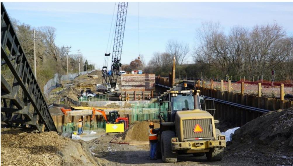
Crews work on abutments for the Minnehaha Creek Bridge. Demolition is completed and sheet wall placement is also in process.
